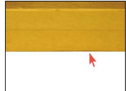
12 If gaps still appear after firm pressure has been applied, use a staple gun. Staple through the tape and wc paper.
